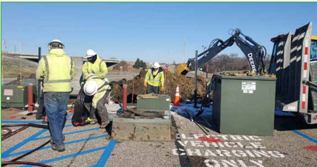
Freeborn-Mower Cooperative Services crews upgraded the electric transformer at the Trails Travel Center, Albert Lea, in preparation for a Fast-Charging EV station being installed by the State of Minnesota Pollution Control Agency.
